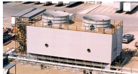
Water is cooled in Sauder's co-generation plant cooling towers
